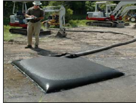
Plate 4.7 Silt bag under inspection
