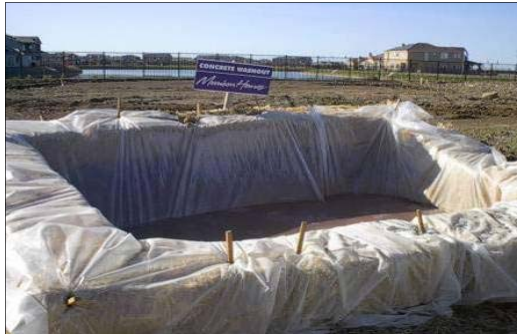
Plate 4.4 Concrete washout area
