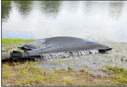
Plate 4.6 Silt Bag with water being pumped through inspection
