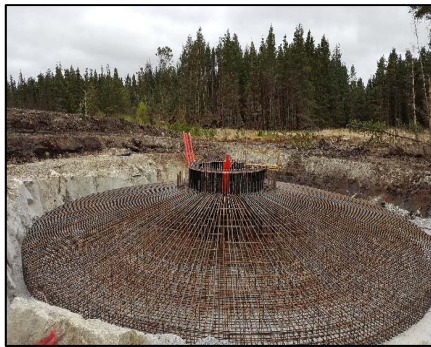
Plate 4.2 Turbine Base 'Anchor Cage'
