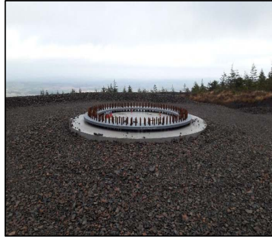
Plate 4.3 Finished turbine base
