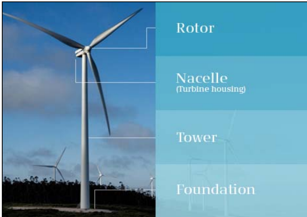
Plate 4.1 Wind turbine components
