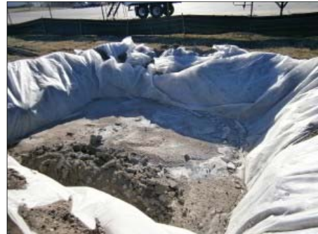
Plate 4.5 Concrete washout area
